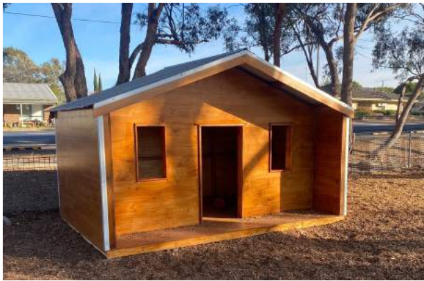
Our cubby house has had the floor and walls replaced
